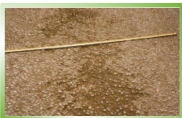
Aggregate Loss / Raveling Segregation
